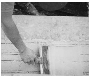
5. Trowel behind the gauge rake using a trowel or tape knife to cover up the gauge rake lines.
