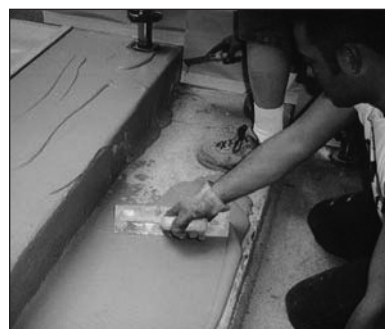
2. Spread the Bond Coat (Resurfacer) over the steps using a trowel and/or wallpaper brush.
