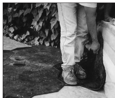
Use the floppy stamp when stamping next to walls or vertical surfaces.
