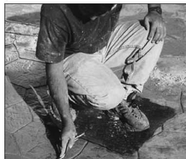
Use a grouting tool to touch-up the grout lines between the two sections, so you can't tell where you stopped and started.
