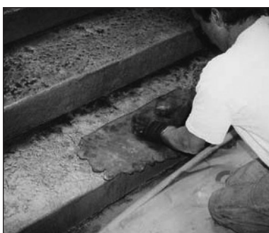
13. Stamp the tops of the steps first by using a texture skin and patting it with your hands to leave the desired impression. Be careful not to pound on the stamps too hard next to the corners so Stamp-Top doesn't lose its bond and fall off the vertical riser.
