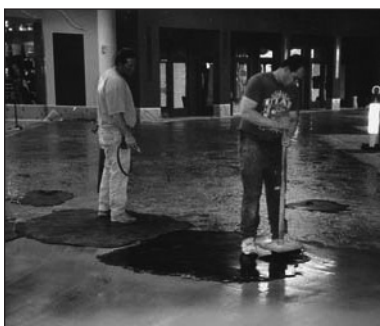
When ready spread a fresh mix next to the 1/4" thick edge where you left off and begin stamping from where you left off.
