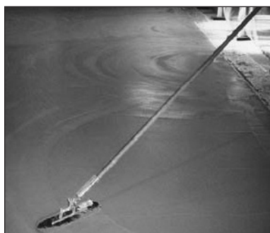
Trowel over the stamping mix with the funny trowel to achieve a smooth finish.
