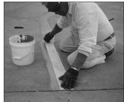
Cover with Elastomeric Basecoat and fabric.
