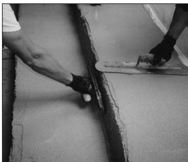
7. Shape and trowel the stamping mix 1/4" thick over the steps as smooth as possible.
