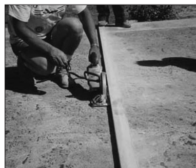
Snap lines and saw cut joints back open.
