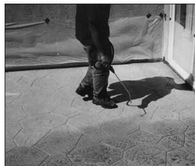
Use the Liquid Release Agent to apply more antiquing, if needed, over the Stamped Concrete Sealer.
