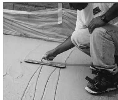
Use a hand trowel and some water to blend two batches together without leaving a seam.
