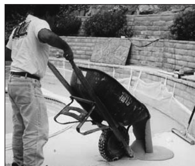
Dump Stamping Mix over Bond Coat.
