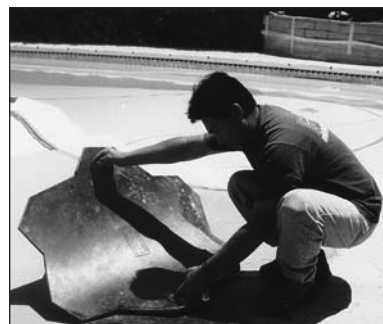
Place more stamps next to the first one so they fit tightly together.
