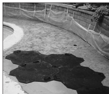
To stop stamping and start again later, cut out around the stamps where you wish to stop stamping.
