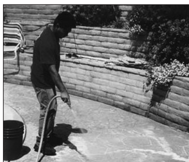
Rinse the surface clean using a water hose or a pressure washer.
