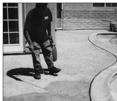
To apply more antiquing, first apply a prime coat of Stamped Concrete Sealer mixed 50/50 with acetone where local laws permit. Apply clear or colored.
