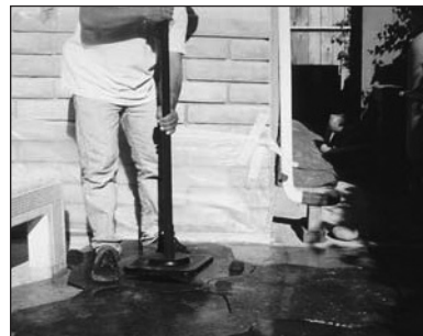
Use the pounder or your feet to imprint the texture from the stamp into the stamping material.
