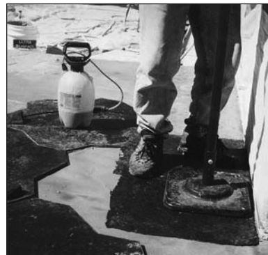
If the stamp mix is firm enough, walk on the texture skins like stepping stones to move around walls imprinting texture.
