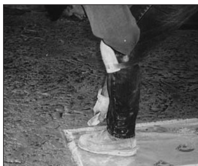
Stamp up to the forms then cut between the forms and the stamp mix using a margin trowel and remove the forms leaving a straight 1/4" thick edge.
