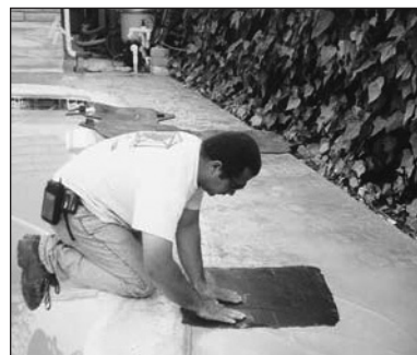
Use texture skins to imprint texture to all the edges and next to walls before stamping.
