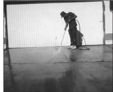
Clean cracks.
