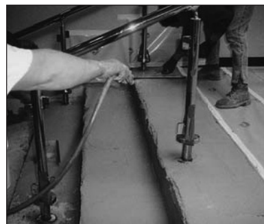
8. Let the mix set up a little firmer, then lightly spray some water and trowel it again.
