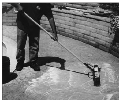
Scrub the surface with a mild detergent and a broom to remove loose antique powder.
