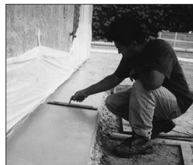
Use a hand trowel to touch-up edges and areas where it is difficult to use a fresno or funny trowel.
