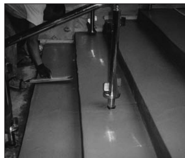
11. After doing the corners, use a hand trowel where needed for touch up.
