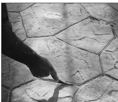
Touch up grout lines where the stamping mix squished up between the stamps.
