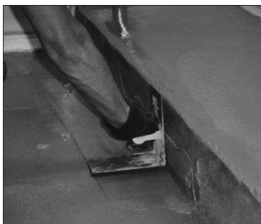
10. Carefully smooth and shape the corners to prepare for the stamping process.
