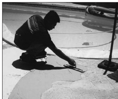
Spread the next mix from where you left off stamping the last section.
