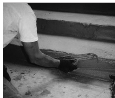
6. Trowel the mix on the top of the steps then up the vertical risers and over the corners.
