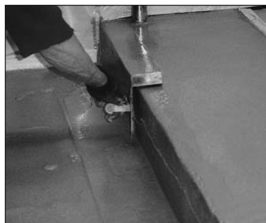
9. After spraying a light fog of water, use some step trowels to shape the step corners.
