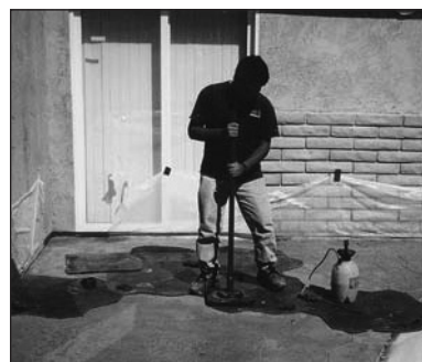
First pound the edges of the stamps, then the middle.
