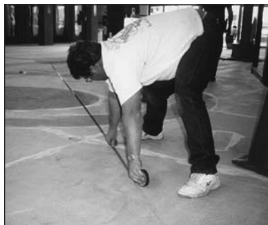
METHOD TWO: Snap a line over the center of a repaired joint or where a saw cut will be made.
