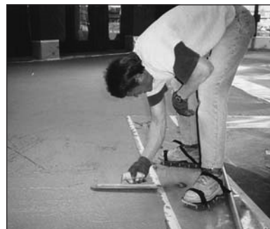
Spread the stamping mix up to the forms and trowel it smooth to the top edge of the form.
