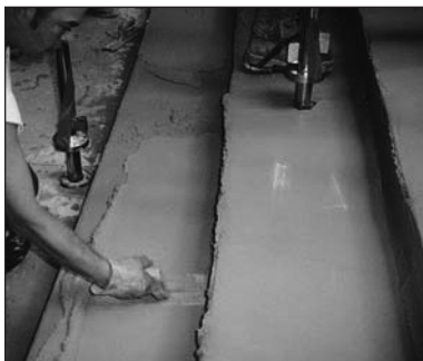
3. Trowel the Stamping Mix over the wet Bond Coat Mix 1/4" thick.
