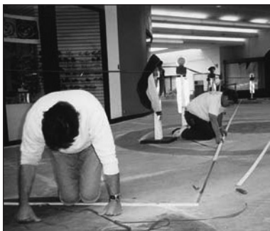
Lay down some 1/4" x 1 1/2" x 8' form strips made out of wood or plastic next to the chalk line using some double sided carpet tape.
