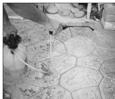
After stamping, spray more Liquid Release Agent with color added to create antique look.
