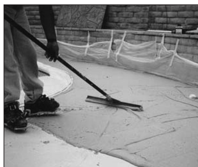
Spread Stamp Mix with Gauge Rake.
