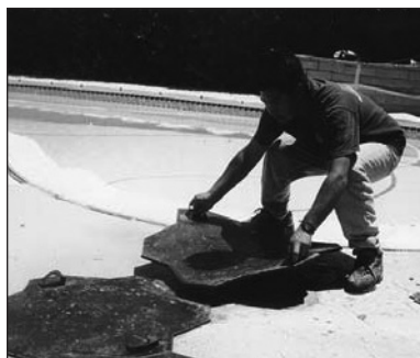
When ready to stamp, fit the stamps over the fresh material next to the finished stamped edge and begin stamping from where you left off.
