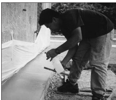
Spray a light coat of water over the surface before troweling for easier workability and to achieve a smoother finish.
