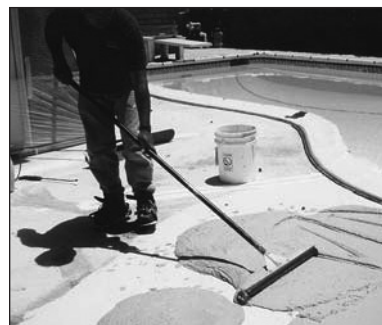
Blend sections together using the Gauge Rake and the Fresno.
