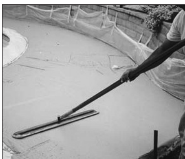
Fresno behind the Gauge Rake.
