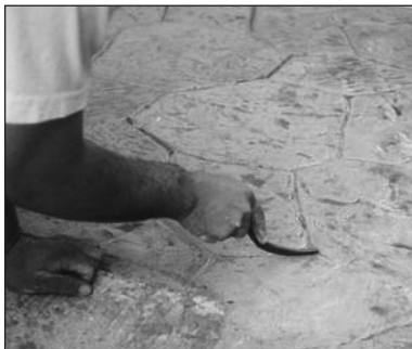
Use touch-up tools to fix grout lines.
