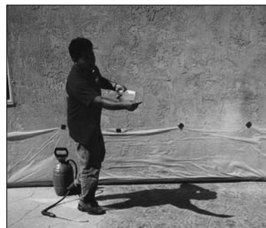
For extra slip resistance, broadcast #80 white aluminum oxide into the Stamped Concrete Sealer.
