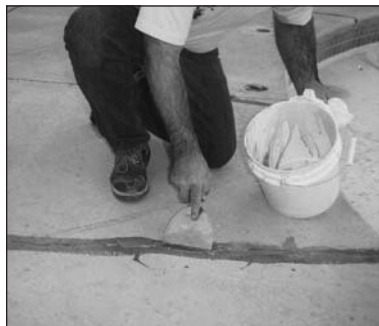
Fill with Epoxy 500 and sand.
