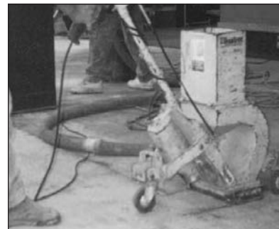
Grind or shotblast for commercial jobs.
