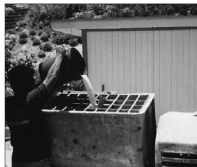
Mix Concrete Solutions Concrete Polymer and water in a mortar mixer. Measure with five gallon buckets.
