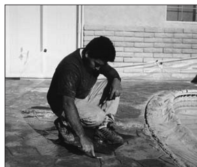
Use the texture skins to walk around on the stamped surface to do touch ups.
