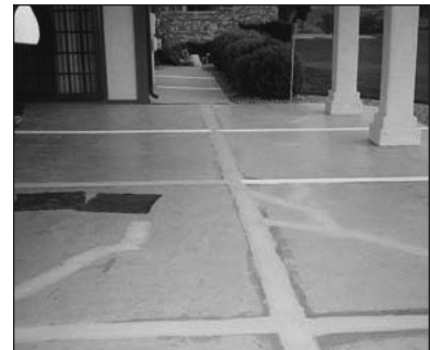
Cover joints with Elastomeric Basecoat and fabric.
