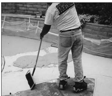
Spread the Bond Coat.
