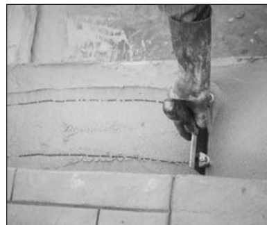
4. Use a hand made gauge rake to leave the material 1/4" thick over the steps.
