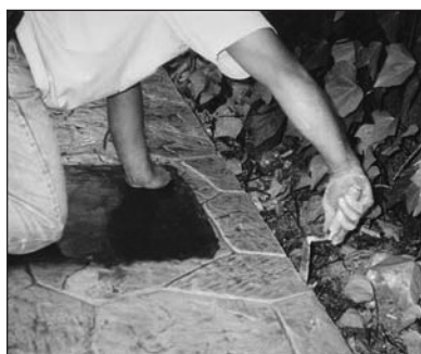
Scrape and detail around all the edges.
