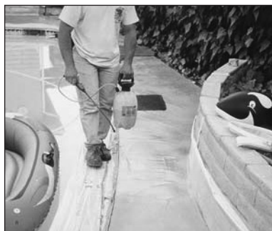
Spray Liquid Release Agent before stamping with texture skins next to walls.
