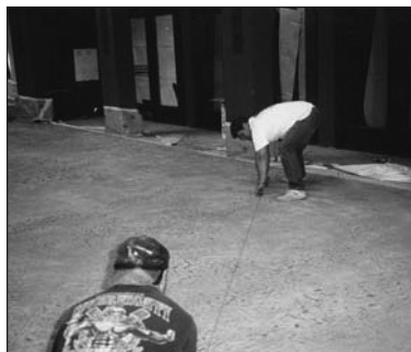
The next day after stamping, snap lines over the center of all the covered expansion joints.
