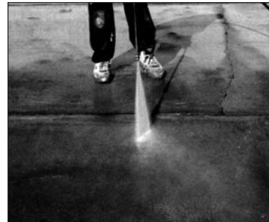
Pressure wash to clean and rinse.
