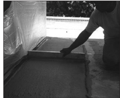
Patch holes, spalls, level or re-pitch.
