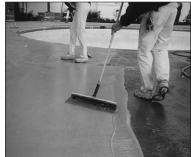
Resurface with Bond Coat.
