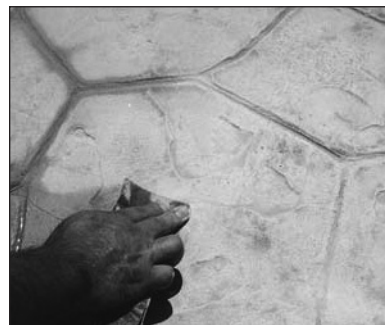
Touch up minor surface blemishes or small surface cracks using #80 – 100 grit sandpaper.
