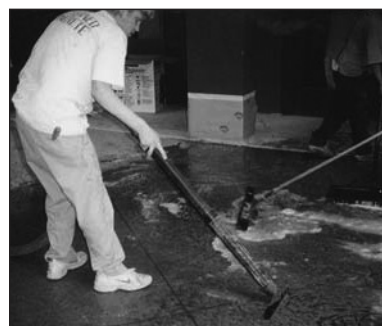
For indoor jobs, a vacuum can be used to remove the rinse water.
