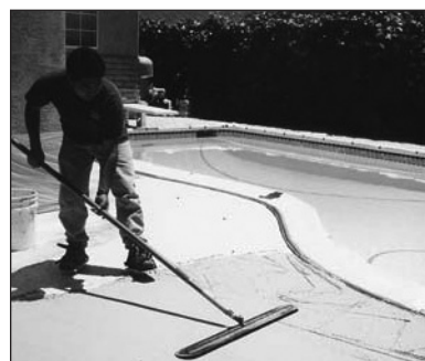
Fresno to fill in Gauge Rake lines.
