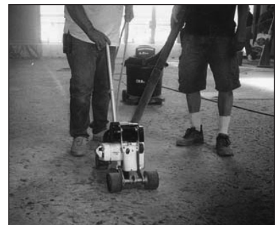
Saw cut joints back open.
