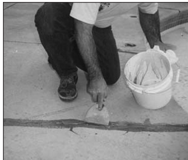
Fill moving joints with Epoxy 500.
