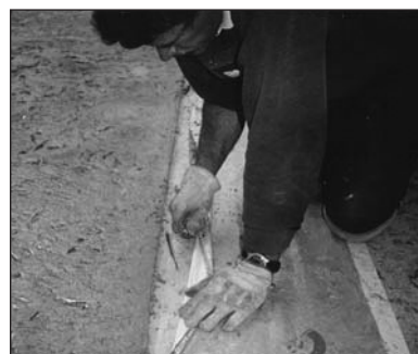
Remove tape next to seam to do any touch ups needed before it dries. Then when dry snap a line over the seam and saw cut.
