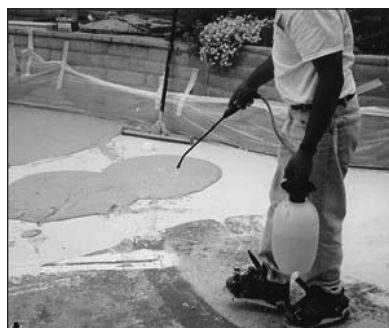
Fog the surface with water.
