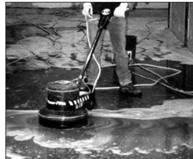
Scrub with detergent and acid wash.
