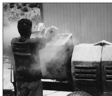
Mix cement, sand and integral color pigment in the mixer or use the pre-mixed bag mixes and Integral Color Paks.
