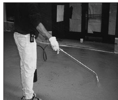
Lightly spray the surface with water prior to using the funny trowel
