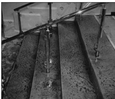
16. Allow the steps to dry then rinse and apply more antiquing using the Antiquing Sealer if needed before applying the Stamped Concrete Sealer.
