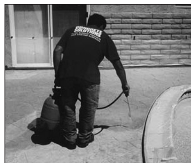
Spray the Stamped Concrete Sealer to even out the color of the stamping application.
