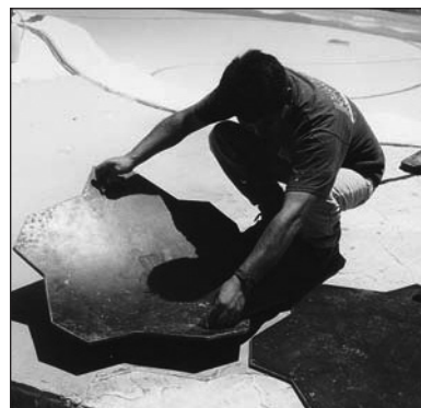
Place the stamps straight down on the stamping material and square with the walls or edges.
