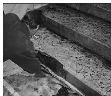
14. Stamp the vertical risers of the steps being careful next to the corners. Use hand tools to create grout lines if stone or tile pattern is desired.
