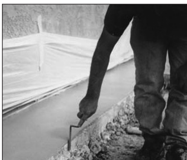
Detail edges using a hand trowel, edger and/or margin trowel while waiting for the funny trowel stage.
