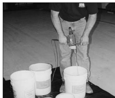
Mix Bond Coat in a five gallon bucket with a 1/2" drill and mixing paddle.
