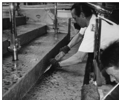
15. Use a chisel and a hammer if needed to gently pound a groove in the inside corner of the steps to leave a finished looking seam line. Use them also to make grout lines if desired.
