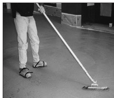
While wearing spiked shoes, funny trowel the surface a section at a time. Lightly spray more water if needed to achieve a smooth finish.
