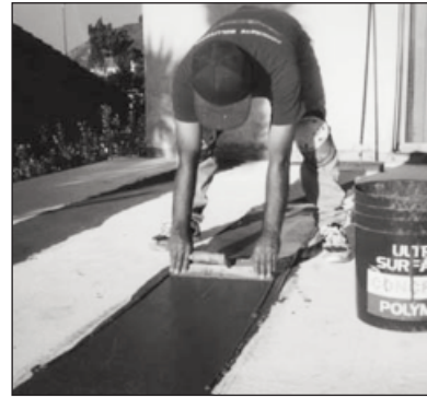
If applying a thin coating system over the fabric, it will be necessary to first patch the seams with Polymer Concrete using a trowel or metal edge squeegee and then apply a Bond Coat (Resurfacer) over the whole surface.
