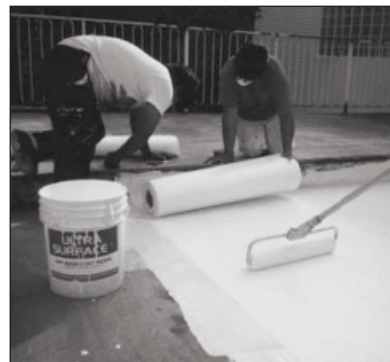
When you reach the end of the deck, cut the fabric with a knife or scissors and start laying the next row.
