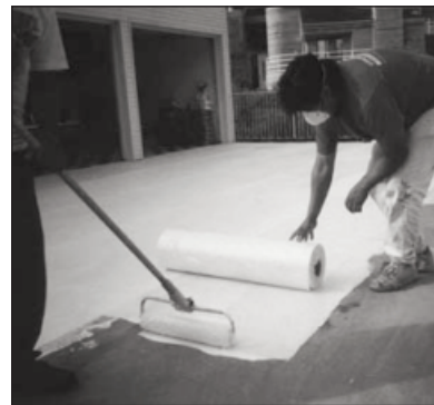
Roll the fabric into the wet Elastomeric Basecoat a few feet at a time.
