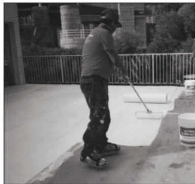
Apply Elastomeric Basecoat ahead of the fabric at 100 sqft per gallon.
