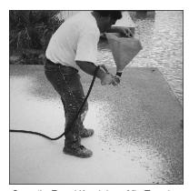
Spray the Trowel Knockdown Mix (Trowel-Top) using a hopper gun sprayer.
