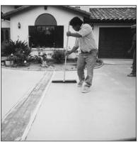
Apply a Fine Broom Finish or Swirl Pattern Finish over the dry Bond Coat (Resurfacer).
