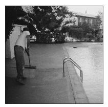
Apply two coats of Concrete Colorcoat undiluted using a 3/4" nap roller.
