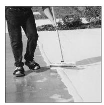
Apply a Bond Coat (Resurfacer) of Polymer Concrete over the surface.
