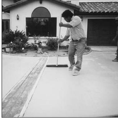
Apply a Fine Broom Finish or Swirl Pattern Finish over the dry Bond Coat (Resurfacer).
