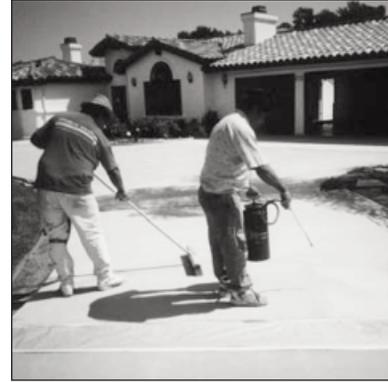
Apply Concrete Colorcoat diluted with 1 – 2 parts of water using a sprayer and a soft broom. When dry, apply a topcoat of Sealcoat 1000.
