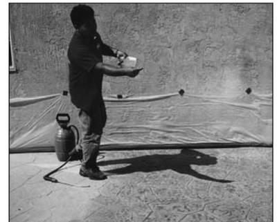
For extra slip resistance, broadcast #80 white aluminum oxide into the Stamped Concrete Sealer.
