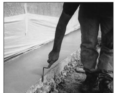
Detail edges using a hand trowel, edger and/or margin trowel while waiting for the funny trowel stage.
