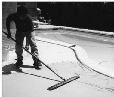
Fresno to fill in gauge rake lines.
