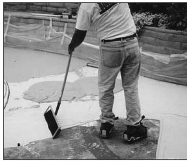
Spread the Bond Coat (Resurfacer).
