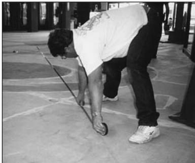
**METHOD TWO:** Snap a line over the center of a repaired joint or where a saw cut will be made.
