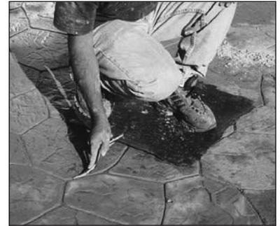
Use a grouting tool to touch-up the grout lines between the two sections, so you can't tell where you stopped and started.
