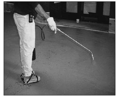
Lightly spray the surface with water prior to using the funny trowel
