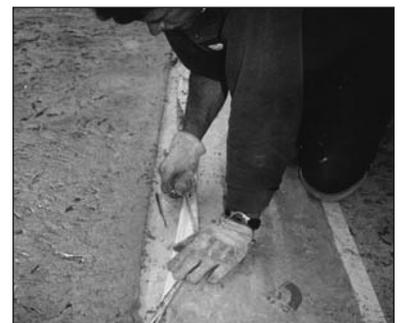
Remove tape next to seam to do any touch ups needed before it dries. Then when dry, snap a line over the seam and saw cut.
