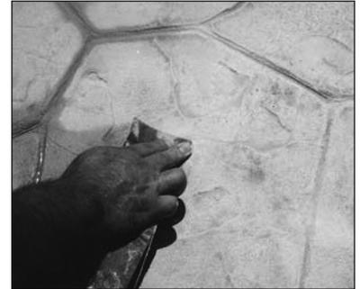
Touch up minor surface blemishes or small surface cracks using #80 – 100 grit sandpaper.
