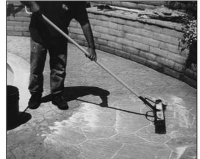
Scrub the surface with a mild detergent and a broom to remove loose antique powder.
