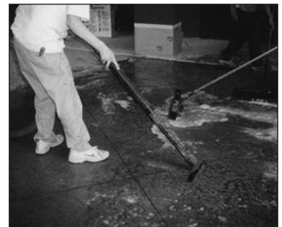
For indoor jobs, a vacuum can be used to remove the rinse water.
