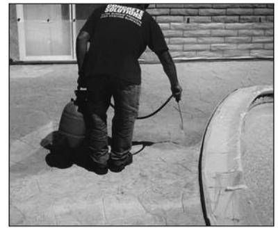
Spray the Stamped Concrete Sealer to even out the color of the stamping application.
