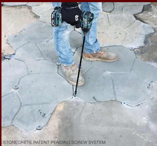
LAYING PATENTED STONECRETE TILES
