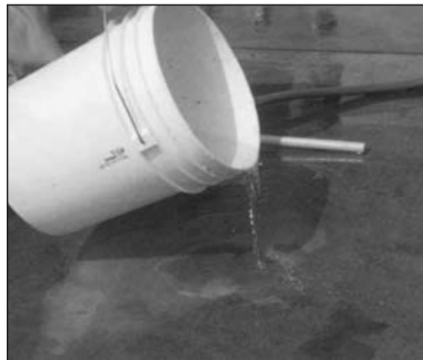
Pour acid solution on dampened floor.
