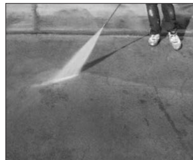
Neutralize, then thoroughly rinse concrete.
