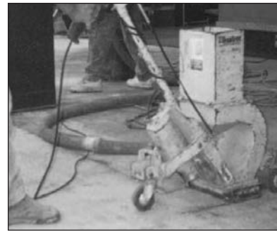
Grind/shotblast to remove paint/sealer
