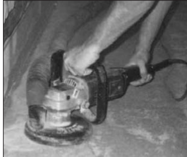
Grind edges and vacuum any residue.
