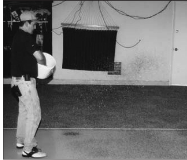
Cover epoxy completely with flakes
