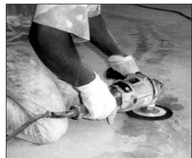
Grind epoxy over crack, smooth with surface.
