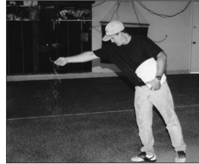
Sprinkle flakes in thin areas or next to edges
