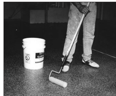
Apply second coat of SB Urethane
