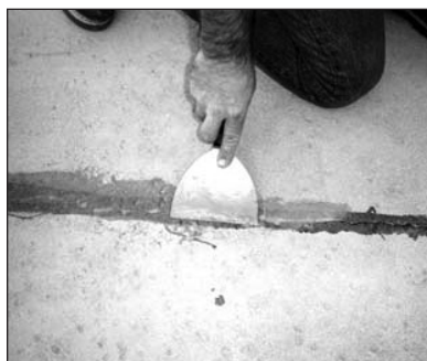
Fill cracks with Epoxy 500 and sand mix
