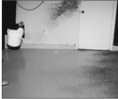
Method 1: When broadcasting with flakes, throw flakes up in the air by hand
