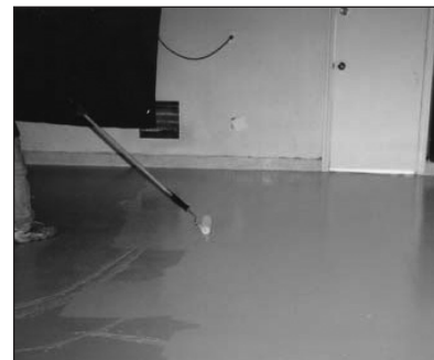
Spread thin with 3/8" nap paint roller
