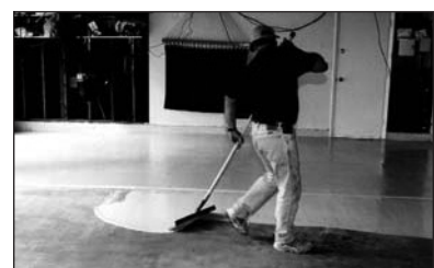
Apply a bond coat (Resurfer) if needed
