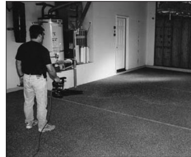
Blow loose flakes to thin areas only if needed
