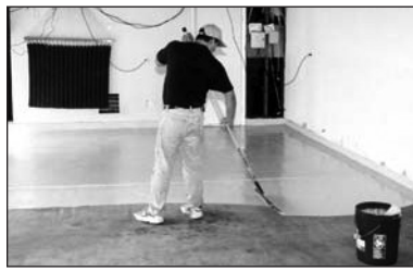
Apply Epoxy 200 with metal squeegee
