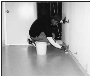
Apply Epoxy 200 Color or WB Epoxy Color to edges
