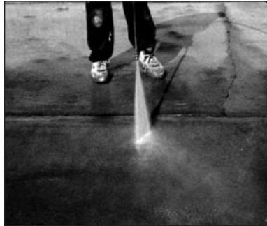
Pressure wash surface to clean and rinse
