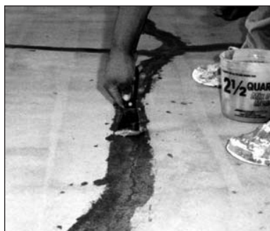
Scrape excess epoxy, leave little above crack
