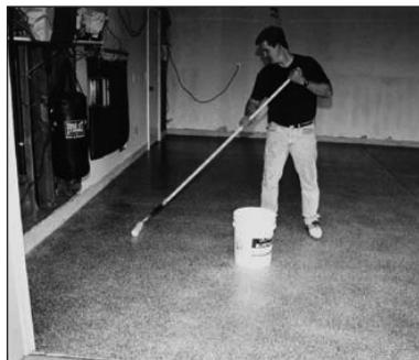
Apply first coat of SB Urethane over flakes
