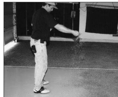
Sprinkle by hand for light to medium coverage
