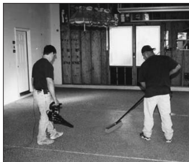
Scrape surface and blow to remove loose flakes or quartz
