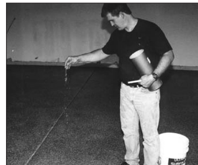
Sprinkle flakes into urethane if needed to even look
