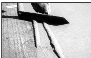
Patch holes or areas needing repair
