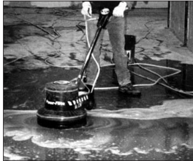
Detergent scrub, acid wash, neutralize
