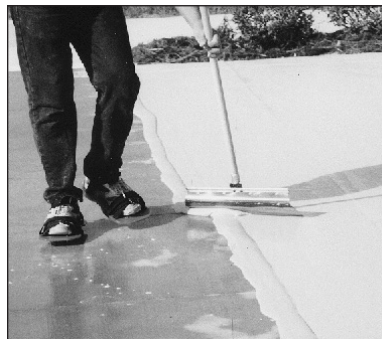
Apply a Bond Coat (Resurfacer) of Polymer Concrete over the surface.
