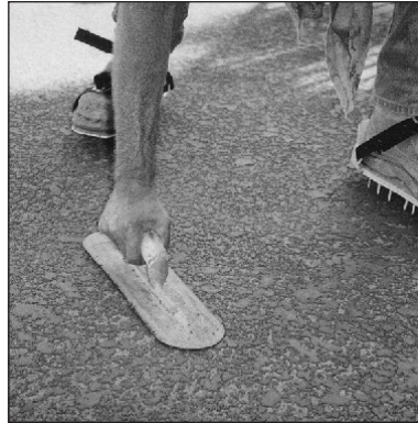
Trowel the sprayed Spray Texture Mix to achieve the desired texture.
