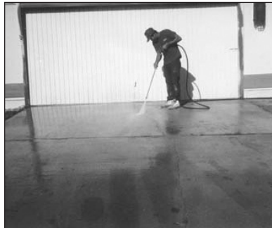
1. Pressure wash cracks.
