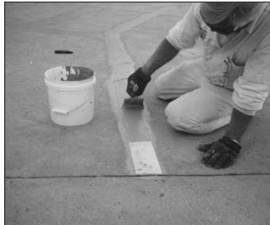
7. Apply Elastomeric Basecoat over fabric.
