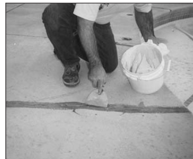
6. Lay crack repair fabric over Elastomeric Basecoat.
