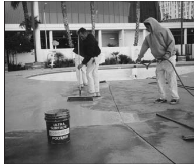
14. Apply a squeegee coat over entire surface.
