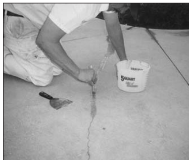
5. Apply Elastomeric Basecoat over Epoxy 500.
