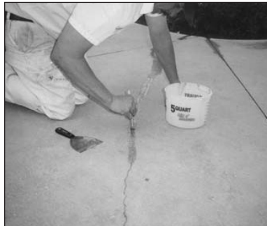
2. Prime with Epoxy 500.
