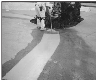
10. Pull the material to a pile.
