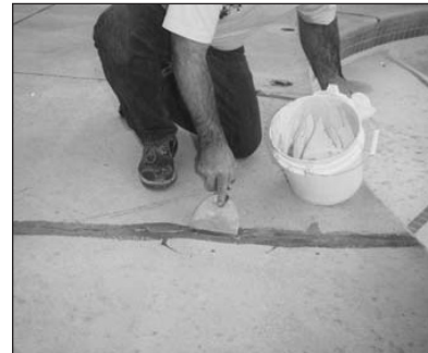
3. Fill with Epoxy 500 sand mix.
