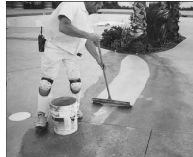
9. Spread patching mix over crack repair.
