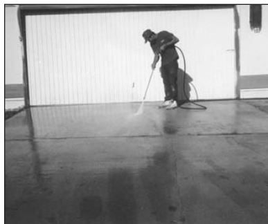
4. Scrape up excess sand mix.
