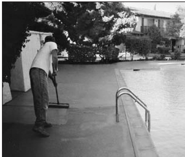
6. Apply Concrete Colorcoat using a paint roller
