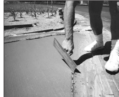
4. Scrape out any material that got in the joints using a trowel or scraper before it dries too hard.
