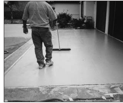
3c. Broom immediately behind the metal squeegee to leave the desired texture.
