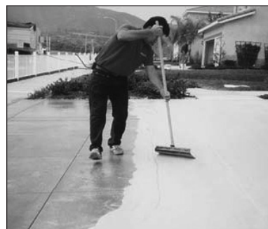
Apply a Bond Coat using a 24" Metal Squeegee.
