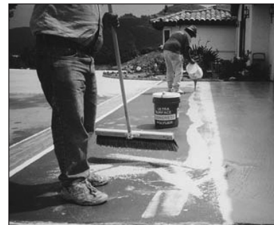
3a. Before the first row of material runs out pour another row on top of it and if necessary spray more water where needed.
