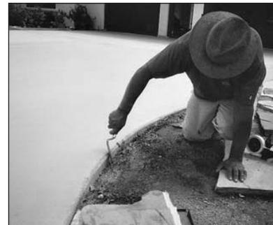
Scrape or brush the vertical edges where the material drips over the sides.
