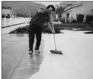
Spread the mix from side to side, in straight rows using a special metal edge squeegee.
