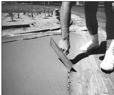
Scrape out any material that got in the joints using a trowel or scraper before it dries.
