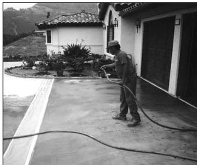
Fog the surface with water where you wish to begin spreading the bond coat/Resurfacer mix.
