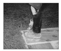
Stamp up to the forms. Then using a margin trowel, cut between the forms and Stamp-Top. Remove the forms leaving a straight 1/4" thick edge.
