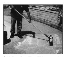
Scrub the surface with a mild detergent and a broom to remove loose antique powder.
