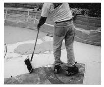
Spread the Bond Coat (Resurfacer).
