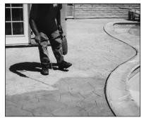
To apply more antiquing, first apply a prime coat of Stamped Concrete Sealer mixed 50/50 with acetone where local laws permit. Apply clear or colored.
