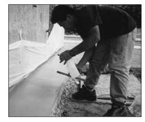
Spray a light coat of water over the surface before troweling for easier workability and to achieve a smoother finish.
