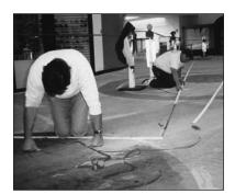
Lay down some 1/4" x 1 1/2" x 8' form strips made out of wood or plastic next to the chalk line using some double sided carpet tape.
