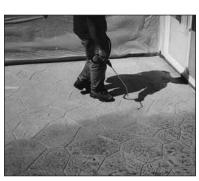
Use the Liquid Release Agent to apply more antiquing, if needed, over the Stamped Concrete Sealer.
