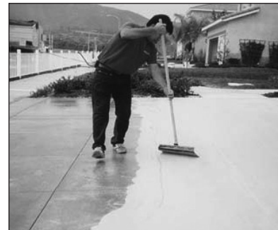
Apply a Bond Coat using a 24" metal edge squeegee.
